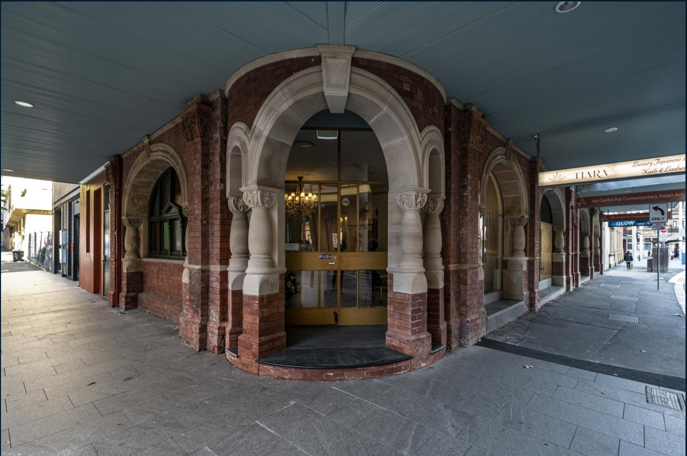
CORPORATION BUILDING, HAY STREET
