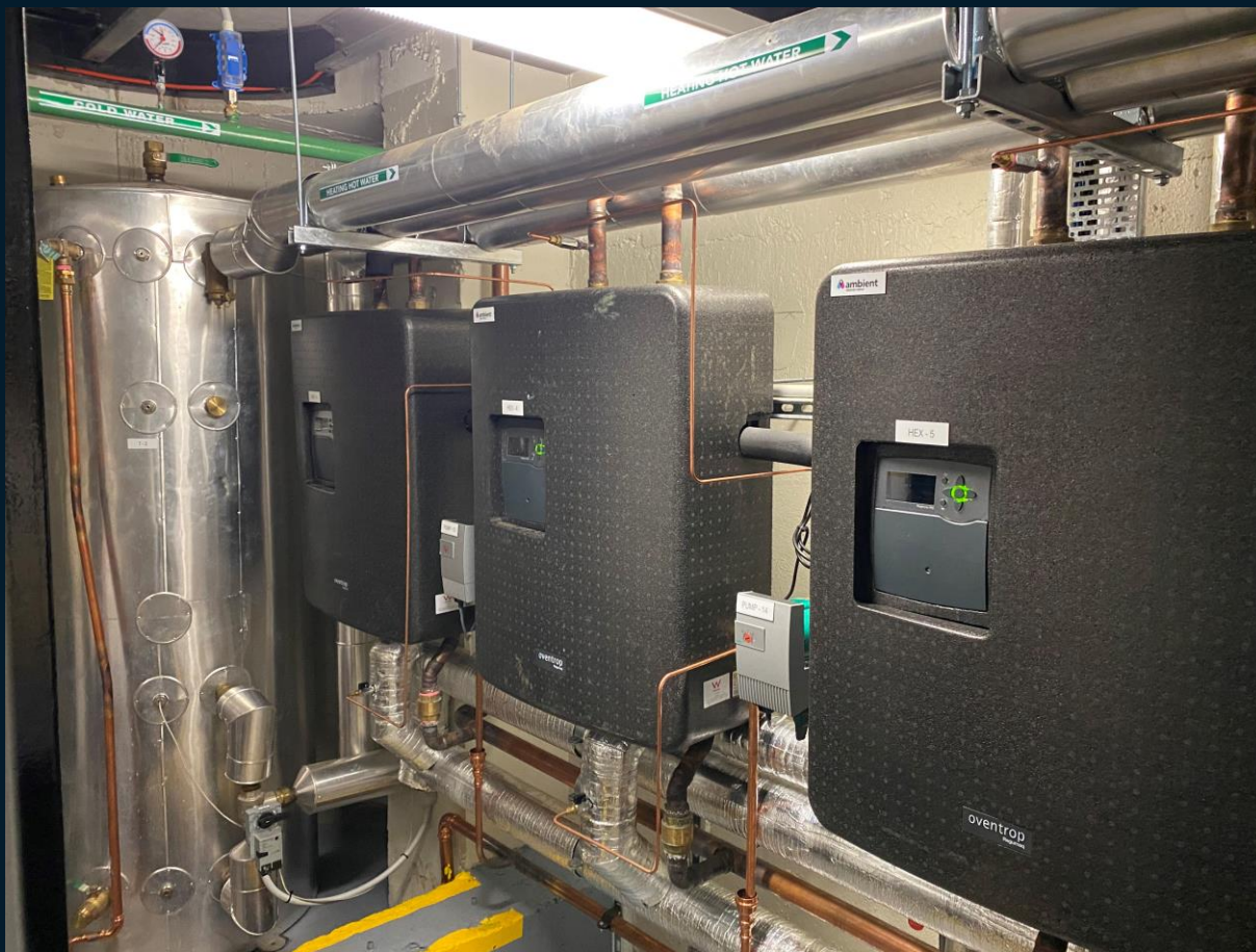
TOWN HALL HOUSE – HOT WATER SYSTEMS UPGRADE
